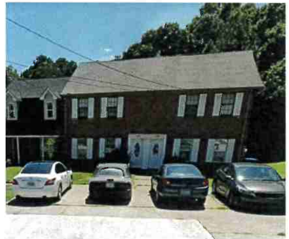
Existing multi-family housing
